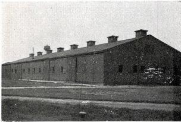
Building No. 68 Engine Repair
